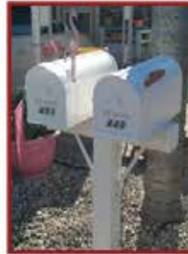
MAIL BOX FRAME REPLACEMENT
