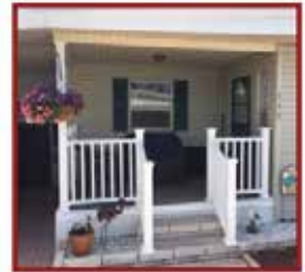
MAX & RENEE'S REMODELED FRONT PORCH WITH RAILINGS
